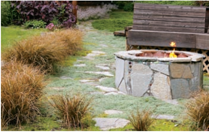
Author's propane firepit with slate flagstone facade and the cap with glass gems and colored stones embedded in the mortar joints
