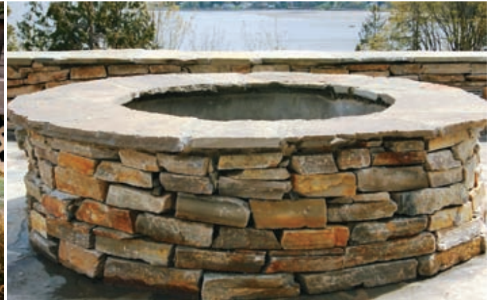
Propane firepit designed by Colleen Miko and built of Goldrush ledgestone with flagstone cap
