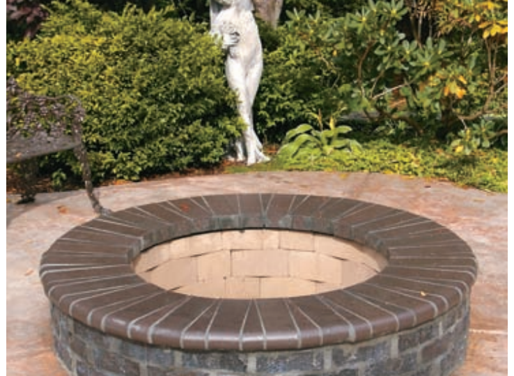
A Woodburning firepit in masonry block with mortared brick facade set in stamped concrete patio
